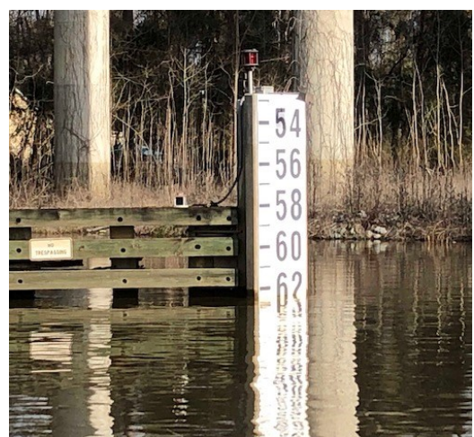
Navigation aid displaying the overhead clearance for a bridge over the ICW in the Myrtle Beach area. Photo by P/C Vicky Jefferis, JN.
